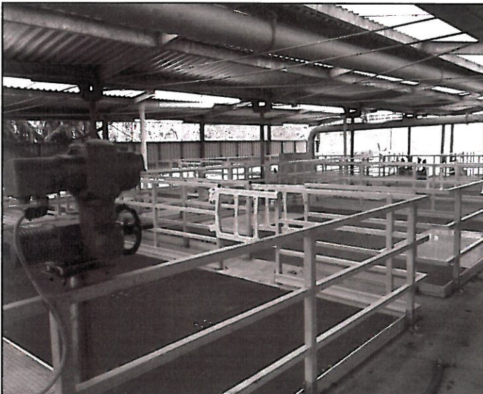
Pictured above are views of the rehabilitated Salmon Creek Treatment Plant Clarifiers, featuring new required safety railing.
