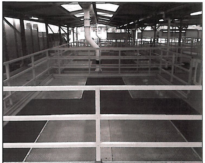
Pictured above are views of the rehabilitated Salmon Creek Treatment Plant Clarifiers, featuring new required safety railing.
