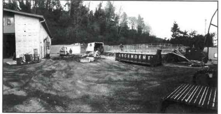
Work has begun at the Salmon Creek Wastewater Treatment Plant
