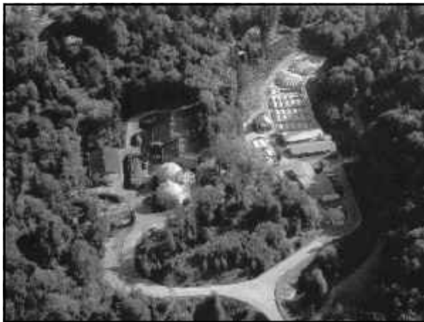
Miller Creek Treatment Plant
