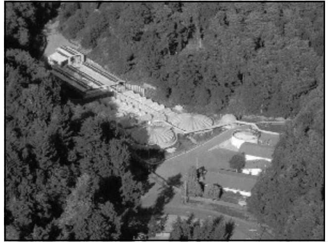
Salmon Creek Treatment Plant
