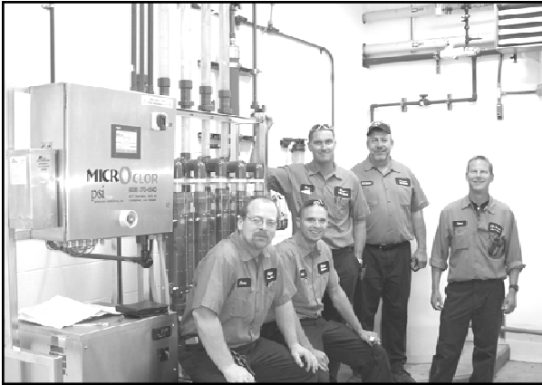
Pictured (L to R) - Plant personnel Shane Cooper, Brett Wittman, Sean Heffen, Michael Grasser and Steve Abegglen in front of the new Onsite Hypochlorite Generating System at the Miller Creek Treatment Plant.
