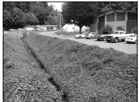
On October 16, volunteers will plant native trees and shrubs on the right bank. District crews will remove the ivy and stabilize the slope prior to the work party.
