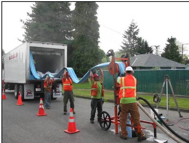
Figure 5. CIPP Rehabilitation
