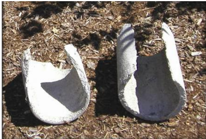
Figure 1. Existing sewer pipe from Chelsea Park Sewer Rehabilitation Project.
