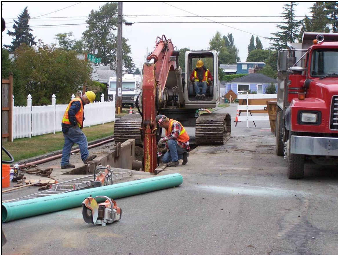
Figure 3. Spot Repair/Pipe Replacement Construction
